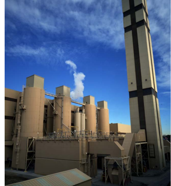
Ogden Energy Fairfax Units 1-4 4 @ 750 TPD Fairfax, VA
